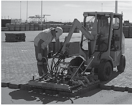
Figure 9. Mechanical installation equipment places concrete pavers rapidly.
