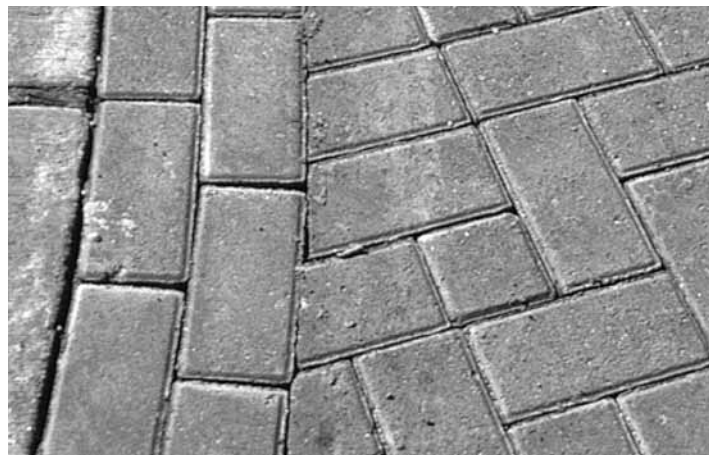
Figure 14. A double row of manually placed pavers along a curb or building provides maneuvering space for the mechanical installation clamp.
