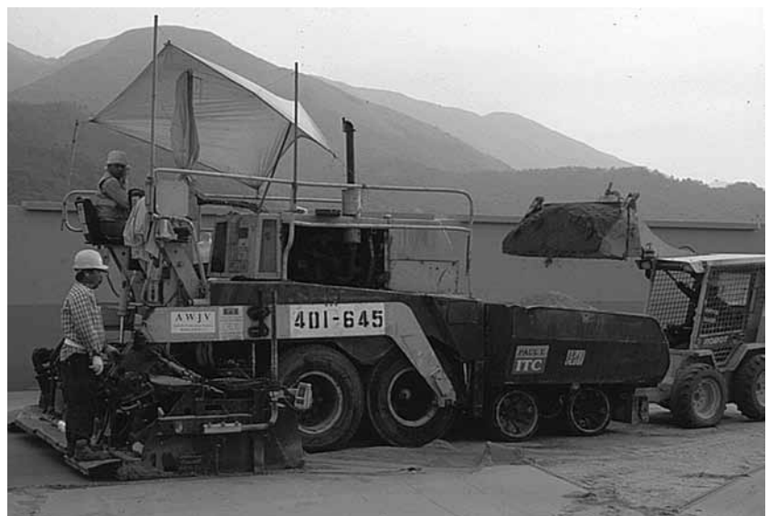
Figure 18. An asphalt spreading machine is modified to evenly and rapidly spread bedding sand.
