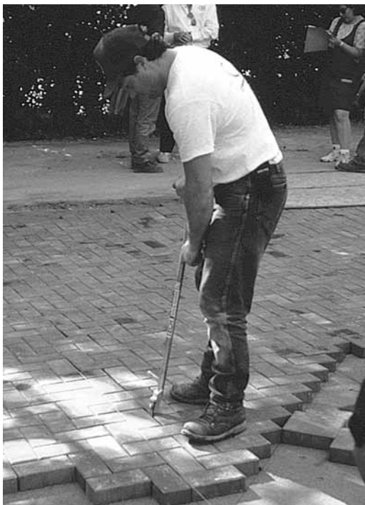
Figure 20. Adjusting joint lines with a pry bar prior to compaction.
