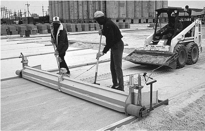
Figure 17. Powered screed bucket accelerates spreading of bedding sand. The width of the bucket can be adjusted.
