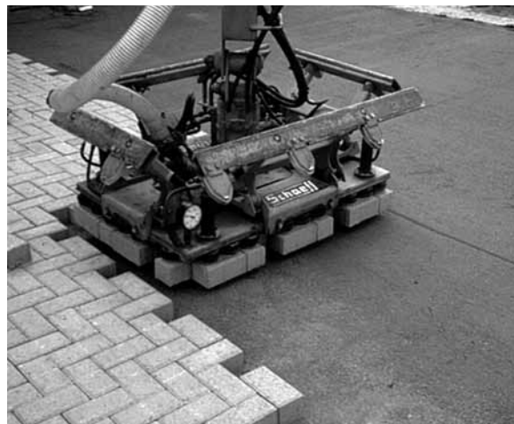
Figure 6. The vacuum head over the paver layer.
