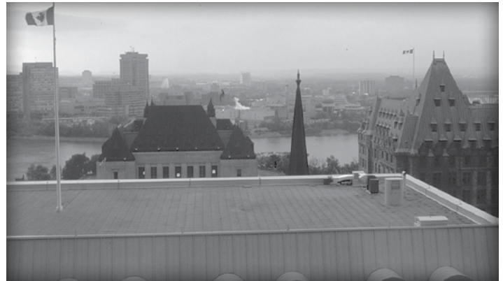
Figure 5. Light colored paving on low-slope roofs reflects light saving on air-conditioning costs while protecting the waterproofing.
