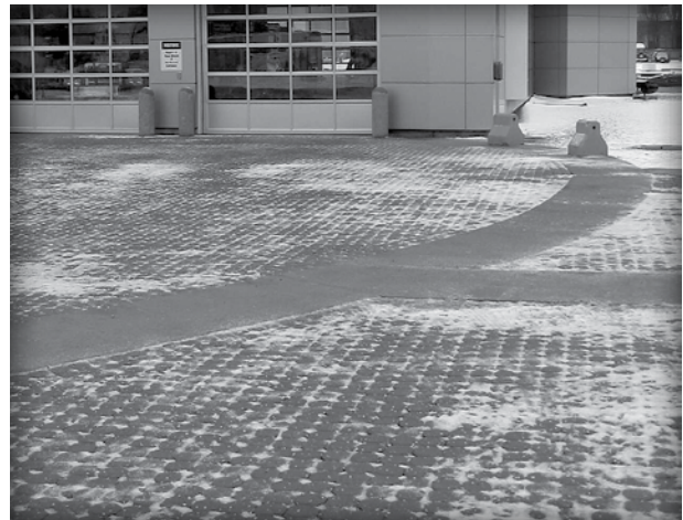
Figure 2. Examples of permeable interlocking concrete pavements for earning LEED® points. The photo on the left shows a hotel entrance in southern California. The photo on the right shows the driveway and parking lot for a fire station in Toronto.
