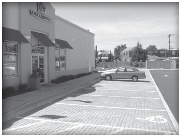
Figure 1. Sustainability for buildings extends to the site with sustainable paving that promotes infiltration and reflects radiant heat from sunlight.
