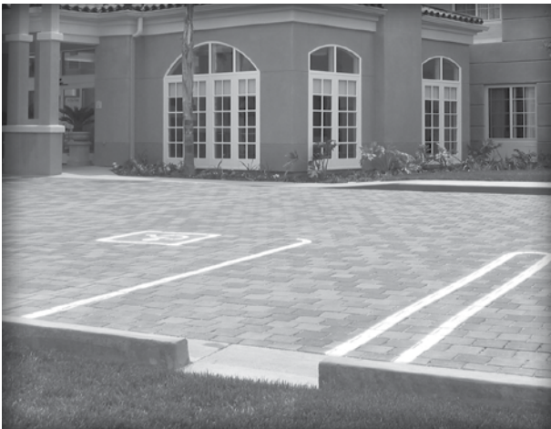
Figure 2. Examples of permeable interlocking concrete pavements for earning LEED® points. The photo on the left shows a hotel entrance in southern California. The photo on the right shows the driveway and parking lot for a fire station in Toronto.
