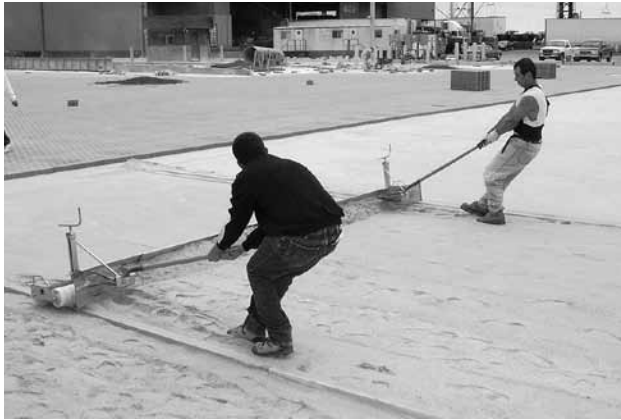
Figure 4. A two-man hand pulled screed
