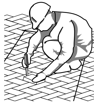
Figure 4. Prying with a screwdriver and pulling the paver out.
