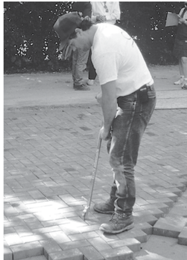
Figure 13 (Left). Adjusting joint spacing and alignment. Figure 14 (Right). Second and final compaction of the pavers. The first compaction occurs after the pavers are placed (no sand in the joints). The second compaction works the sand on pavers into the joints. This process causes the pavers to interlock.
