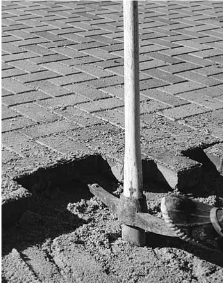
Figure 6. Prying out the remaining pavers
