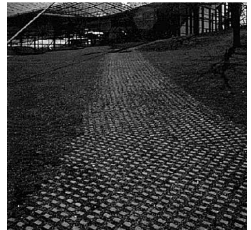
Figure 7. Service access lane
