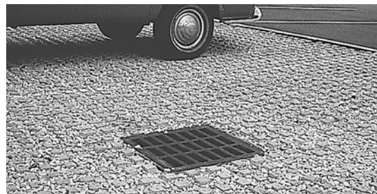
Figure 18. Concrete grids with aggregate in the openings
