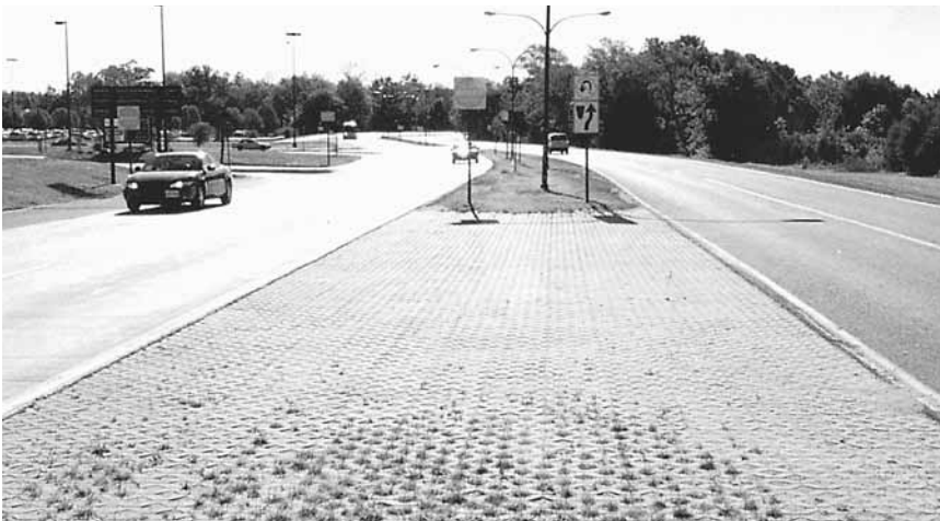
Figure 6. Roadway median crossover
