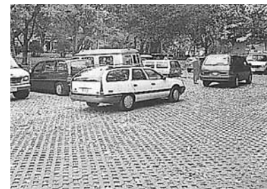
Figure 16. A parking lot with a dense-graded, crushed stone base.
