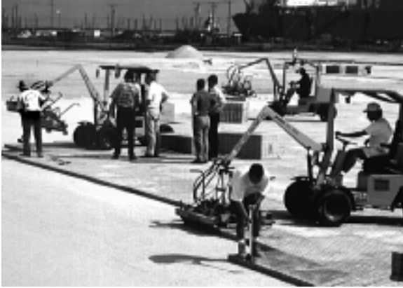
Figure 9. Mechanical installation equipment places concrete pavers rapidly.
