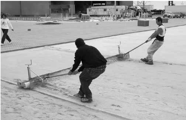
Figure 4. A two-man hand pulled screed
