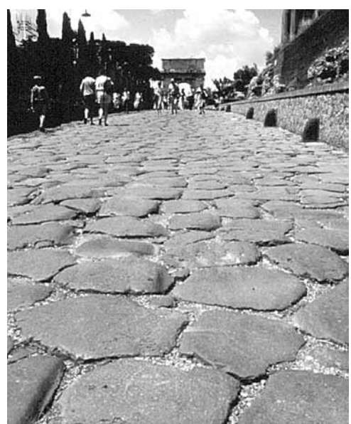
Figure 1. The Roman Appian Way: early interlocking pavement
