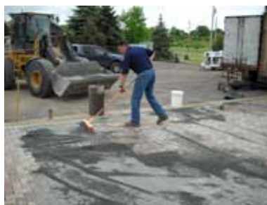
Filling joints with AquaStone5 (5mm clean)
