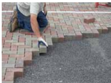
Laying Perma Piazza pavers on setting bed
