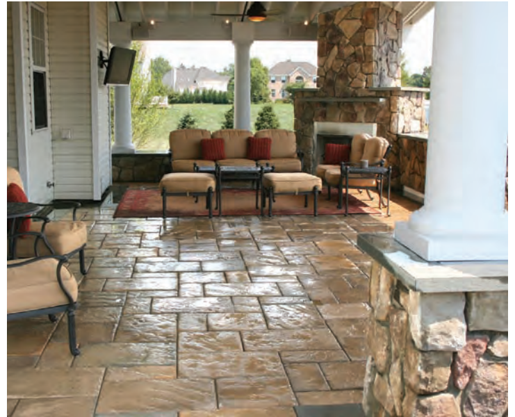
Steps leading to a backyard patio are created using stamped concrete with a natural stone border. Photo courtesy of Carrero & Sons Concrete and Construction
