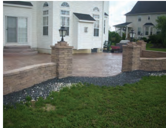
This spacious patio, constructed of stamped concrete, leaves the homeowners plenty of room for entertaining and enjoying the outdoors. Photo courtesy of Carrero & Sons Concrete and Construction
